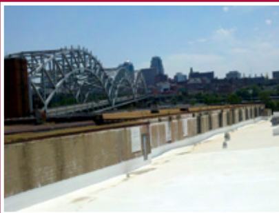
After applying GacoFlex S-20 the roof surface is smooth and defect-free
